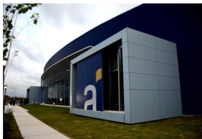
There are 33 data centers around the world like the Antel building and only four are located in South America
